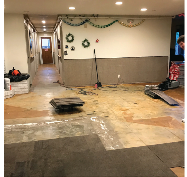
Floor remodeling in progress
