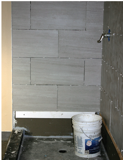
Shower room remodeling in progress
